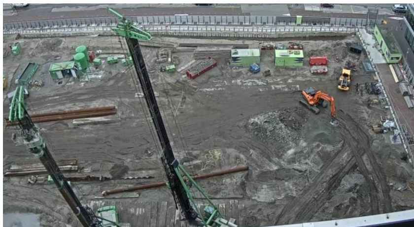
Figure 1 Construction site with positions of foundation piles
