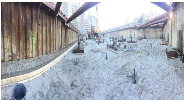
Photo 6 Excavation of the building pit
