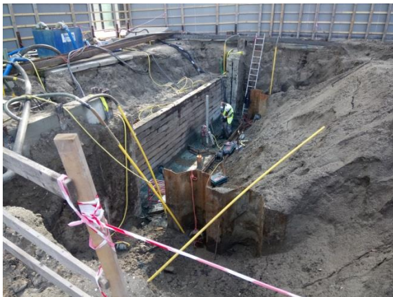
Photo 3 New Babylon tunnel preparation
