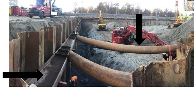
Photo 7 Girders (arrow left) and punch frame (arrow right) in the corner Rijnstraat / Bezuidenhoutseweg
