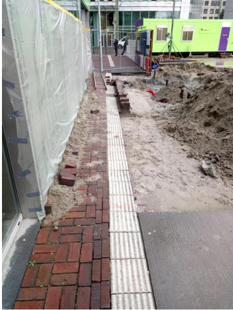
Photo 9 Removing the walkway
