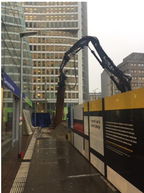
Photo 10 Drilling of the obstacles
