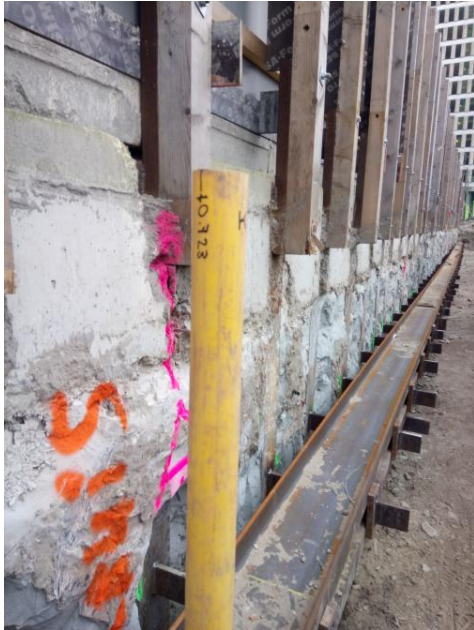
Photo 5 Monitoring well in the building pit
