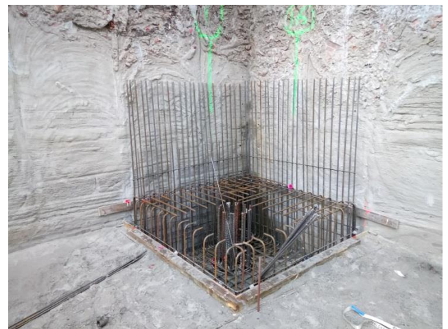
Photo 8 Concrete reinforcement of the foundation piles
