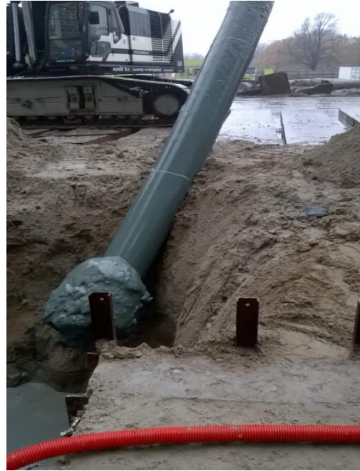
Photo 11 Removed foundation pile
