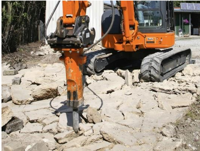
Photo 2. Example of crane hammer that will demolish the concrete
