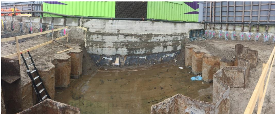
Photo 1. Current situation of the New Babylon Tunnel
