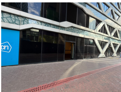
Photo 7 – correct entrance to the moving area, next to Albert Heijn
