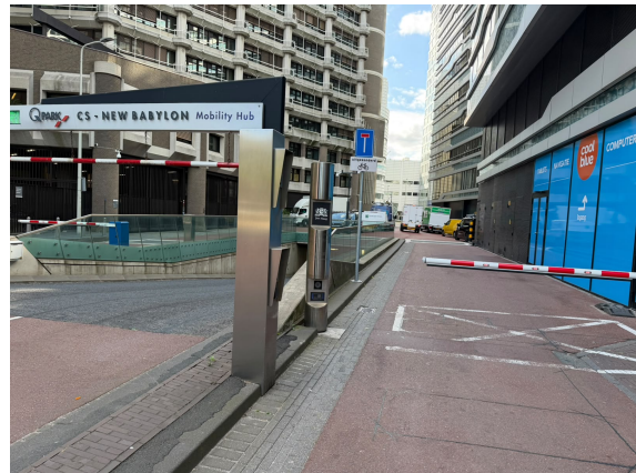
Photo 2 – barriers House of Representatives, intercom. Between Q-Park CS - NEW BABYLON Mobility Hub (alternative, no trailers, max. 2.05 m) and Coolblue
